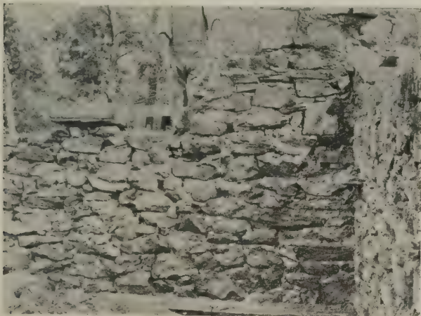
Fig. 3. Inside face of wall shown in Fig. 2
